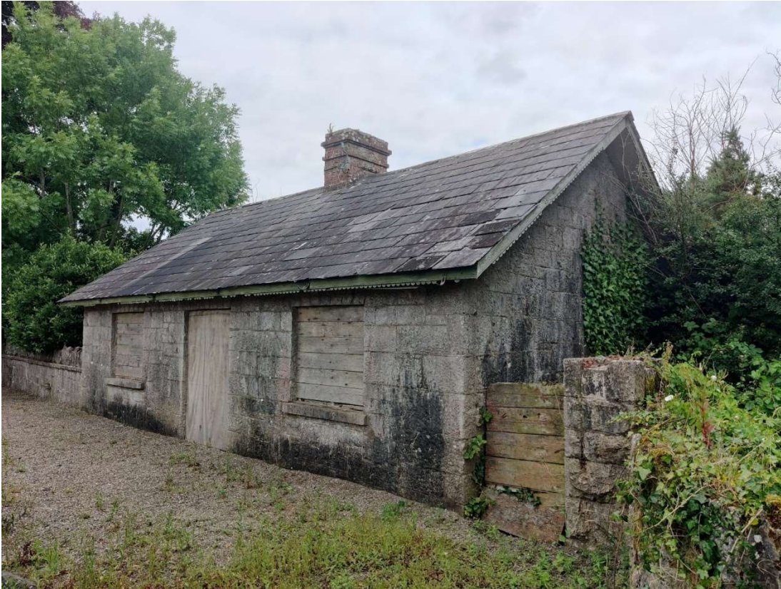
Figure 12-19: Block and Mortar Bungalow
