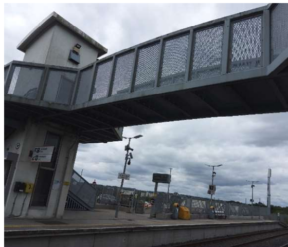
Figure 12-25: Steel Type Bridge
