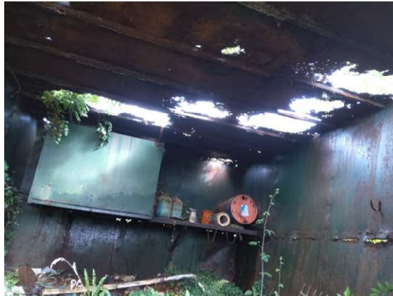
Figure 12-23: Roof Gap in Shed
