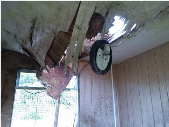
Figure 12-22: Roof Gap in Prefab
