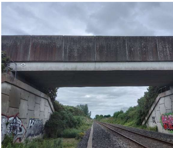
Figure 12-24: Concrete Beam Type Bridge
