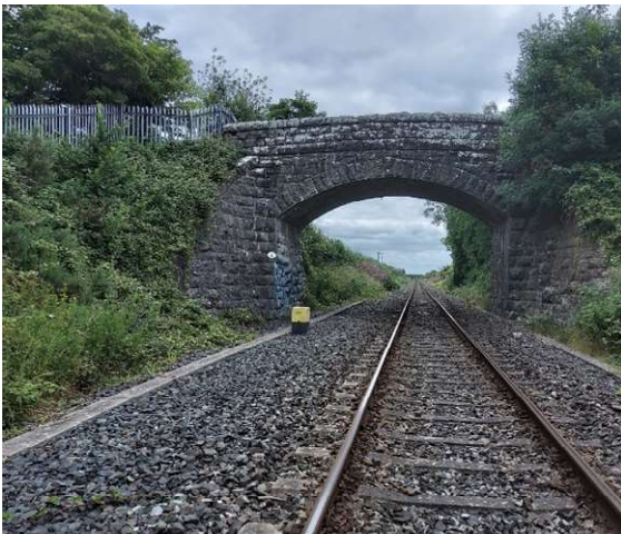
Figure 12-26: Brick Type Bridge
