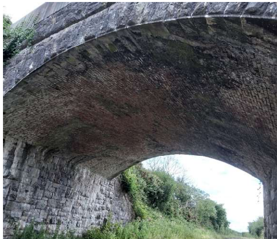
Figure 12-27: View of Brick Bridge Arch
